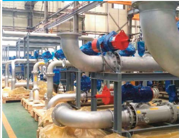
Front Pipe Skid
