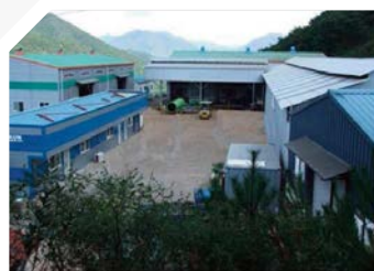
TSA Coating Factory
