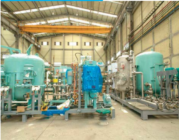
Fresh Water Supply Plant
